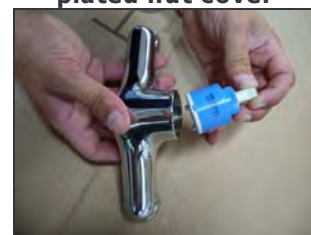
6 - remove the cartridge
