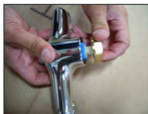
5 - undo the brass nut
