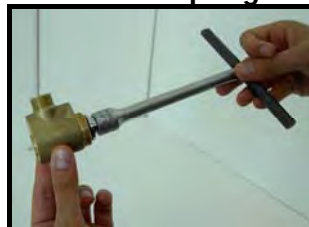
5 - undo the cartridge
