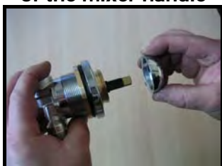
17 - undo the chromium-plated nut cover
