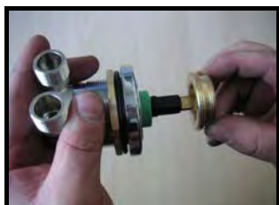
18 - undo the brass nut
