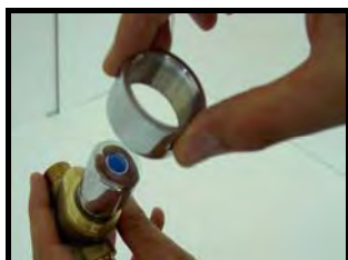
1 - undo the outer ring nut
